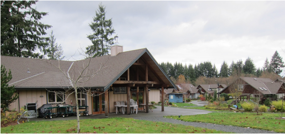
Image 4 Common house in the foreground, private duplexes in the background, Creekside Commons Courtney BC
