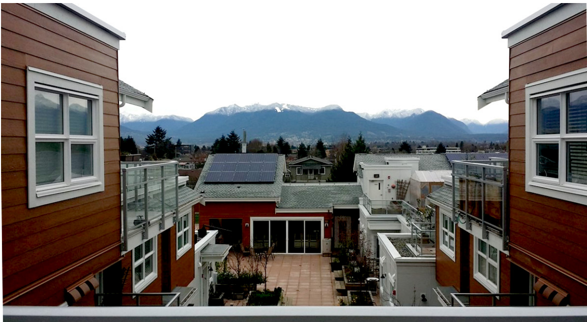
Image 7 View of Courtyard and common house (beneath solar panels), Vancouver Cohousing, Vancouver BC
