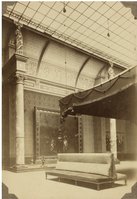
Figure 4. The canopy was installed at the Rembrandt Gallery because the public complained that it was hard to see the obscured painting under the skylight. Anonymous, Rembrandtzaal gezien vanuit het noordoosten , c. 1886-1886, photographic paper, Rijksmuseum, Amsterdam, RMA-SSA-F-00041-1. Image Source: Rijksmuseum.
