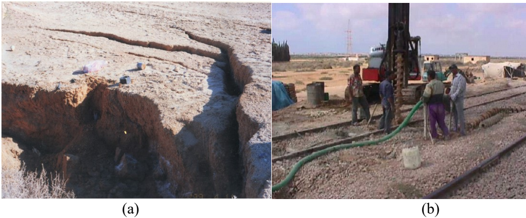
Fig. 1.2. (a) Sinkholes developed nearby the railway line; (b) Filling the voids by grouting as soil treatment (Sakr et al., 2008)
