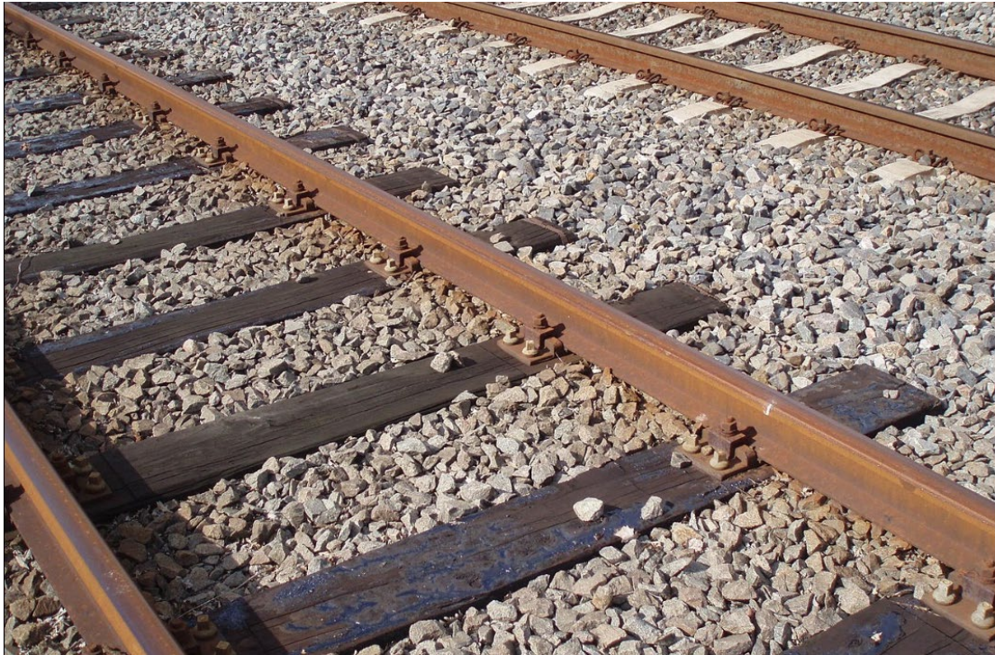
Figure 3. 3. Timber sleepers (LooiNL 2007)
