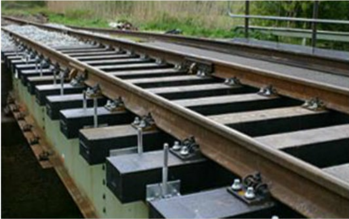
Figure 3. 4. Steel railway sleepers (AGICO GROUP 2020)
