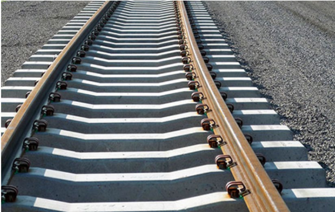
Figure 3. 5. Mono block concrete sleepers (AGICO GROUP 2020)
