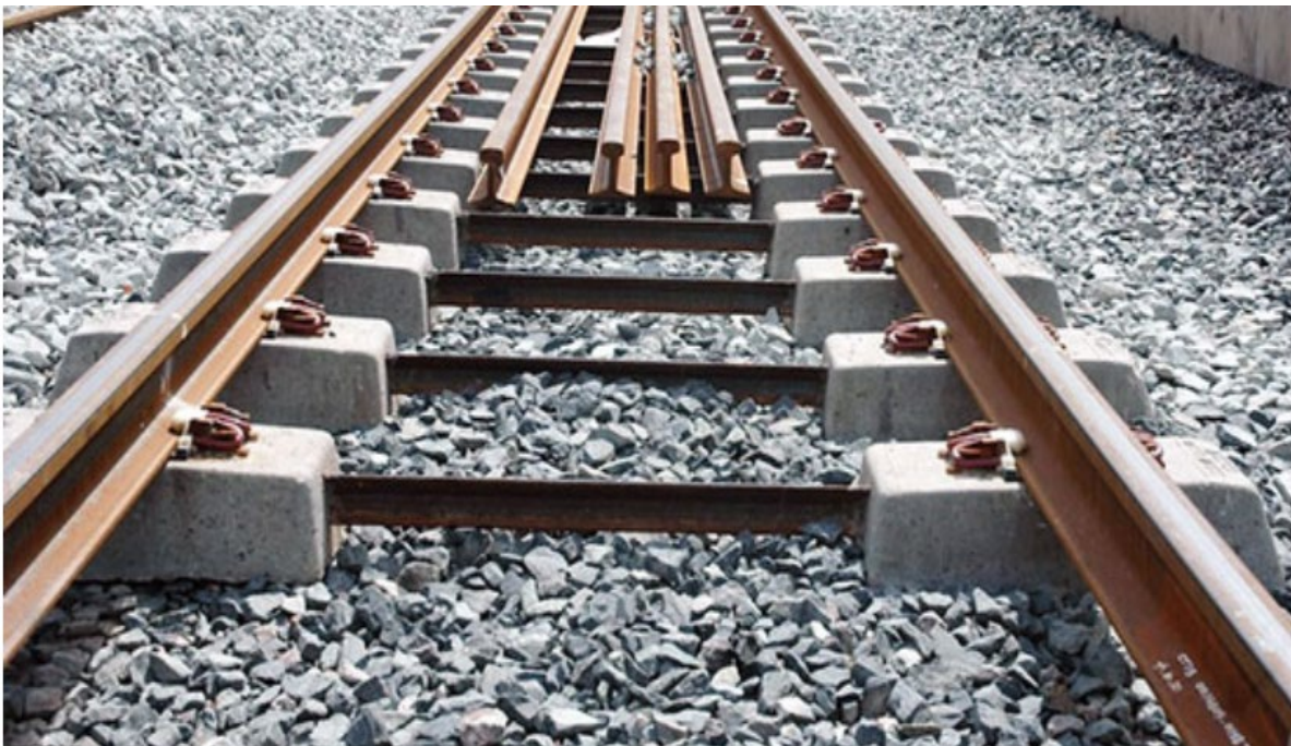
Figure 3. 7. Twin-block concrete sleepers (AGICO GROUP 2020)
