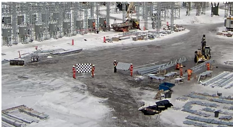
Figure 4-12 Example of image frames with two check boards for calibration
