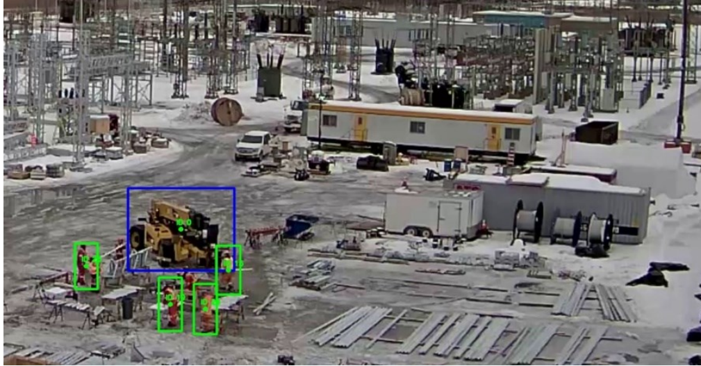
Figure 4-10 An example of workers close to the equipment
