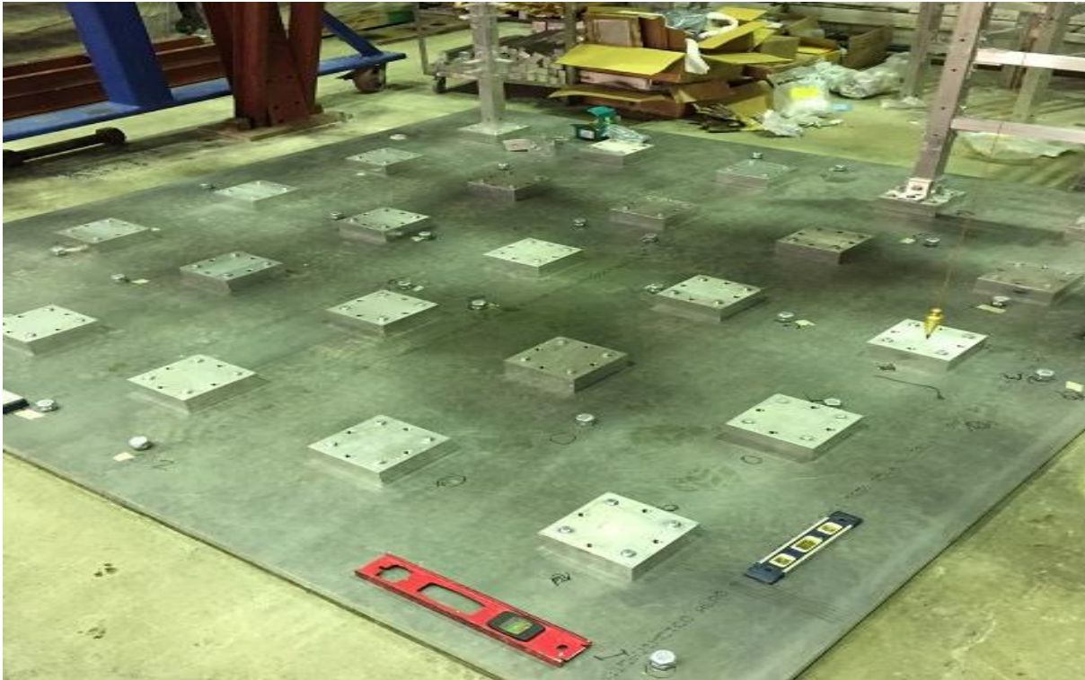
Figure 3.6 Base leveling
