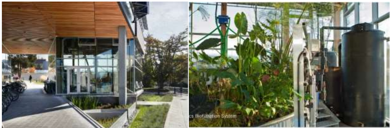
Figure 7.19. Solar aquatics filtration system of the CIRS (2011) - © Peter Busby of Perkins and Will
