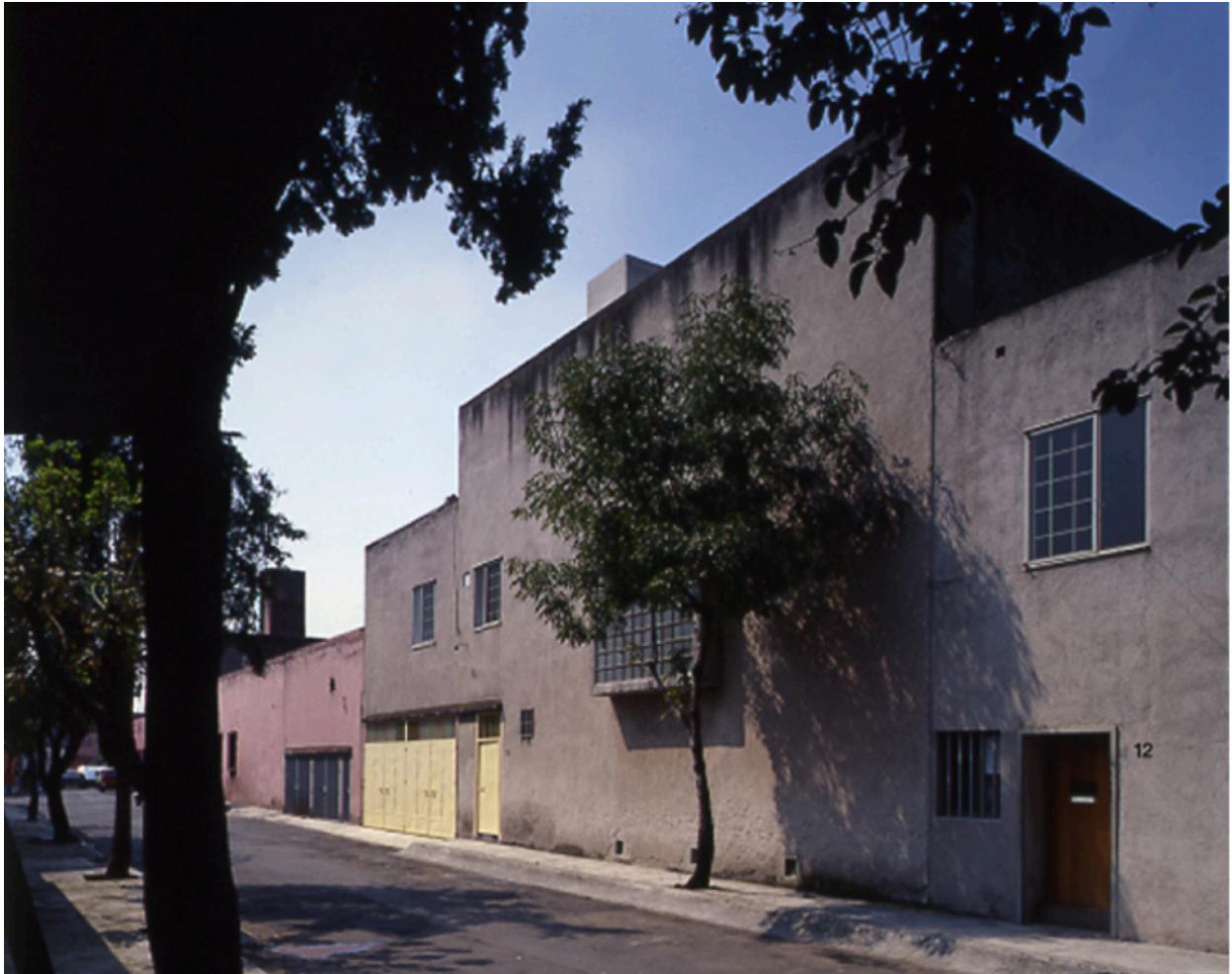
Figure 1- Building's façade Mexico City. Unknown Photographer. Image source: http://www.-casaluisbarragan.org/lacasa.html
