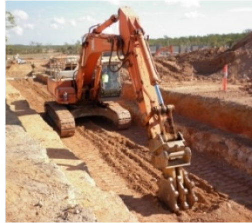
(b) Compaction wheel attached to Hoe
