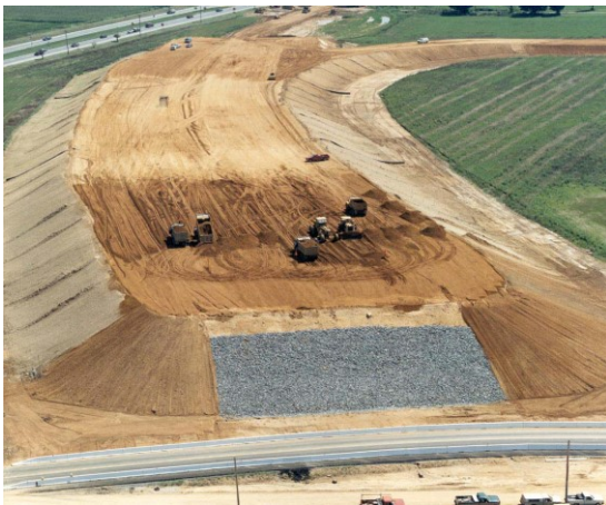
(a) Road Embankment Construction.
