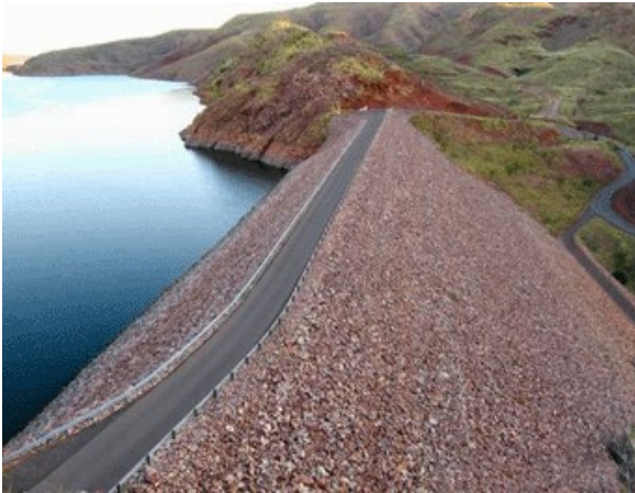
(c) Earth Dam.
