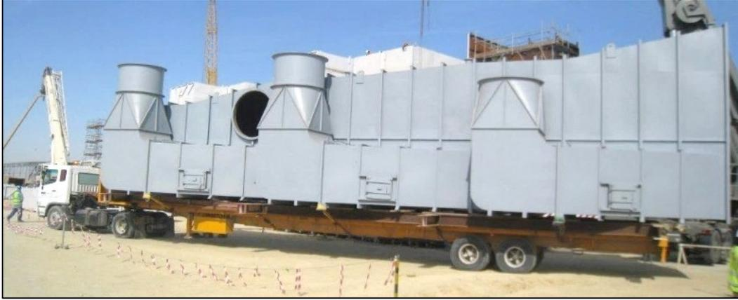
Fig. 4.1: A duct segment with stiffened plate walls being delivered in an industrial project [courtesy of fives Inc.]
