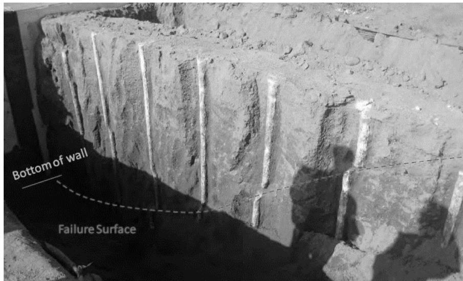
Fig. 2-16 Path of the failure surface after (Stewart et al., 2011, p. 74).
