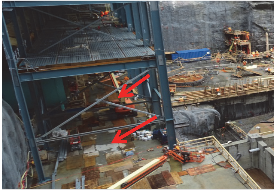
Figure 5-2 As-built tagged site picture at day 20
