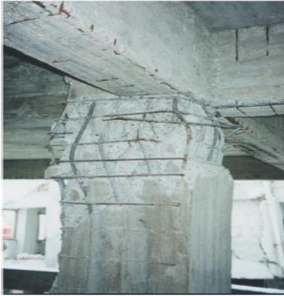
Figure 1.1. Damaged column due to an earthquake [Ilki \(2006\)](#).
