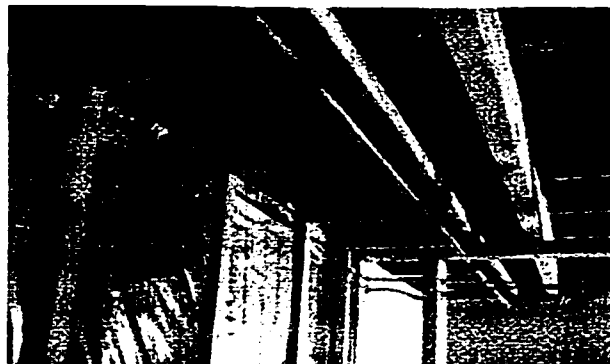
Figure 2.10. View of the cavity L5, which has lateral leakage all along lateral wall. The furring on top of the polyethylene sheet leaves a space for air leakage behind gypsum board. At bottom right of picture, the interior partition can be seen. Leakage occurs through that partition as well.
