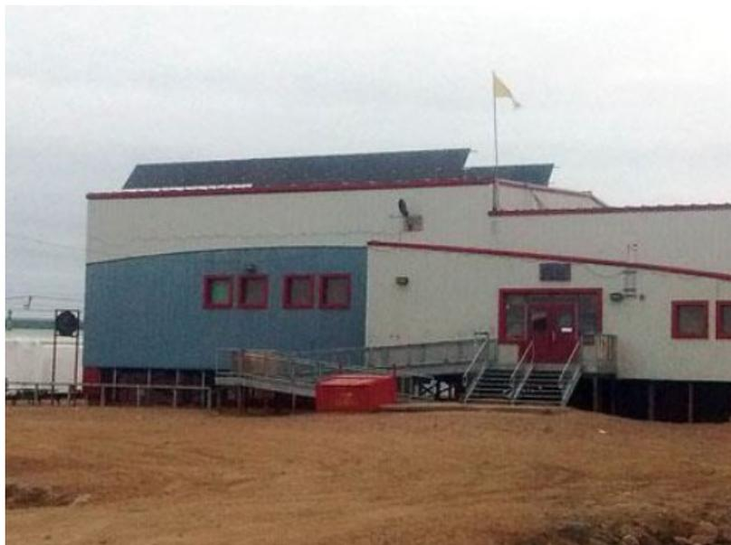
Figure 2.8 Pond Inlet PV system install on roof of building to avoid vandalism (Rogers, 2018).
