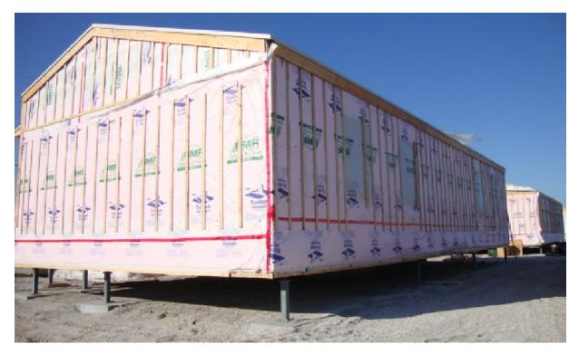
Figure 3.1 Vertical furring strips presently used on standard Nunavik housing construction. (Photo taken by author)
