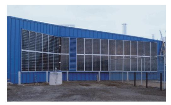
Figure 2.17 Kuujjuaq, QC LEED certified airport with 6.3kW PV array (Matrix Energy, 2007).
