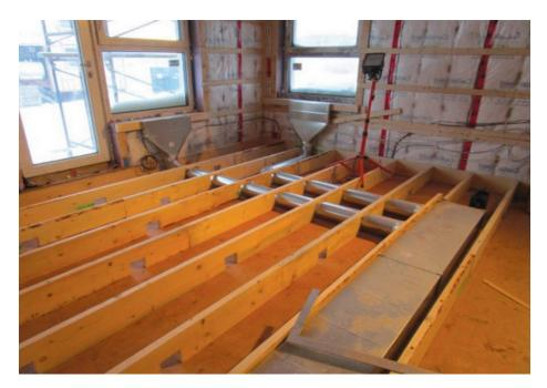
Figure 2.15 NHP subfloor ventilation ducts (SHQ, 2020)
