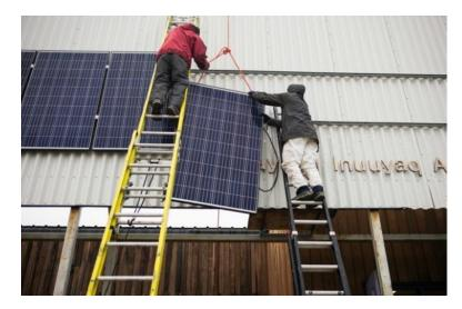
Figure 2.7 Solar array being applied to the façade of the Clyde River community center (Rogers, 2018).
