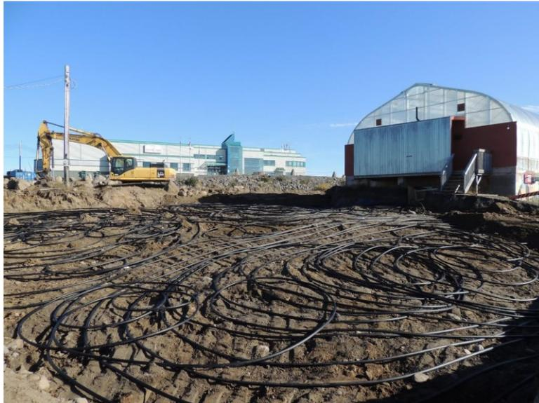
Figure 2.21 Kuujjuaq solar/ geothermal pool heater (Giordano & Raymond, 2020).
