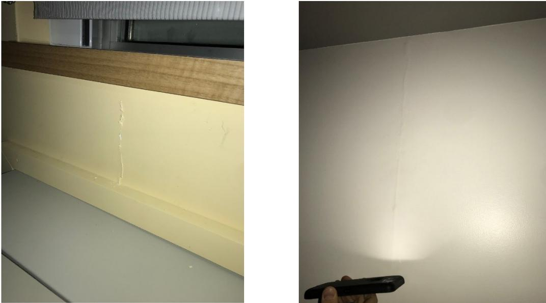
Figure 3-5: Sample of actual damages (cracks) on prefabricated individual modules caused by the transportation-induced forces
