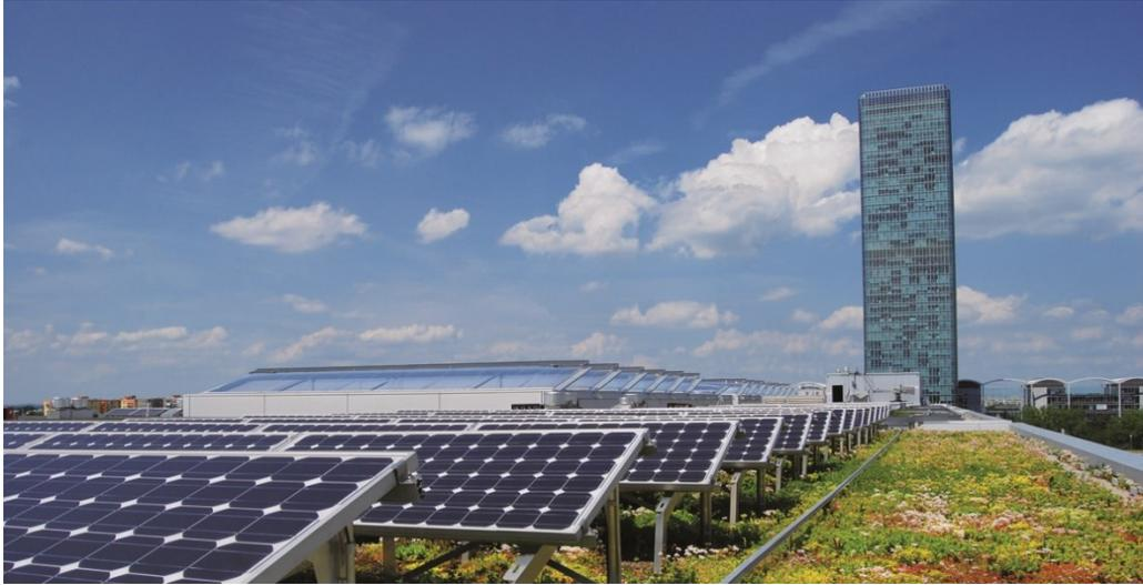
Figure 3.12 An example of Biosolar Roof
