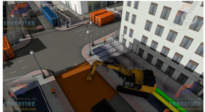
(b) Trench excavation
