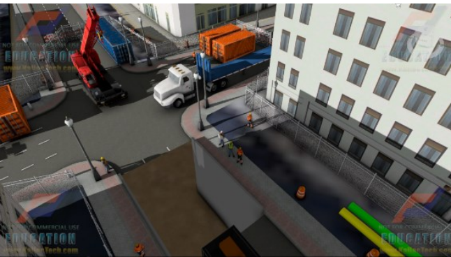
(c) Installation of trench shoring system
