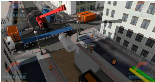
(e) Placing the tunnel section
