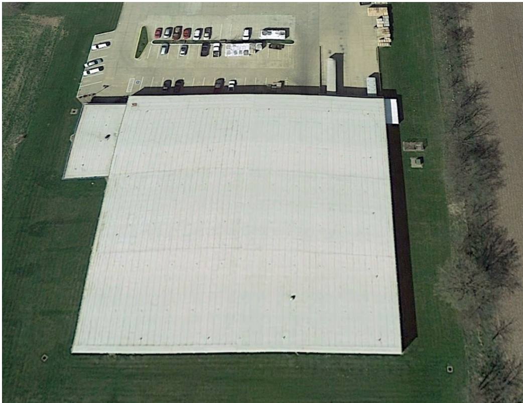
Figure 13: The experimental building of Duro-Last Roofing Inc. in Iowa (Google Earth).
