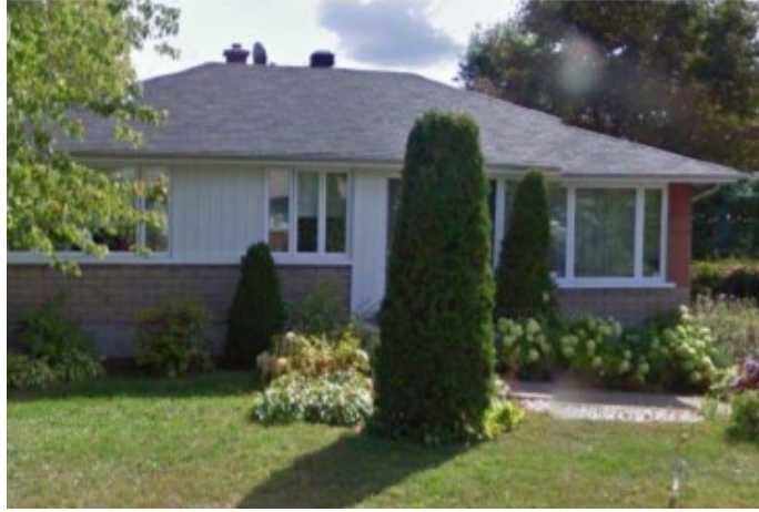
Figure 4-8: Experimental building used in the case study of Task 3
