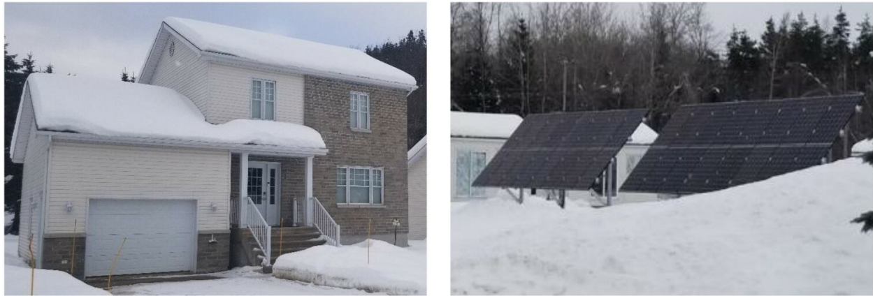
Figure 1.5 EHBE, Shawinigan, Québec [15].
