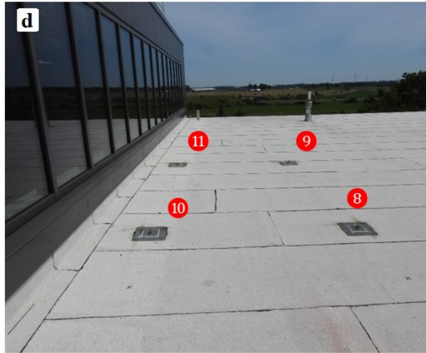
Figure 2: Photos of pressure taps on the lower and upper roofs
