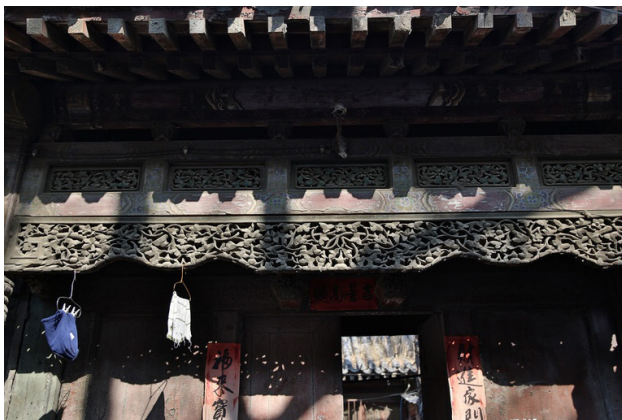
Decorations on the west second entry door in Rongyuanzhai (Bai, 2015)
