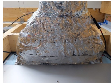
Figure 4.2.18: BIPV/T manifold after additional layer of reflective insulation
