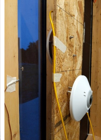
Figure 6.2.15: SGR4 pyrometer facing indoor surface for Method B2
