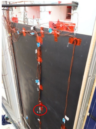
Figure 3.1.6: Sensor setup for the air cavity and back pan, the HMP50 relative humidity sensor (circled in red) is positioned near the center of the wall cavity and fixed with sheathing tape.
