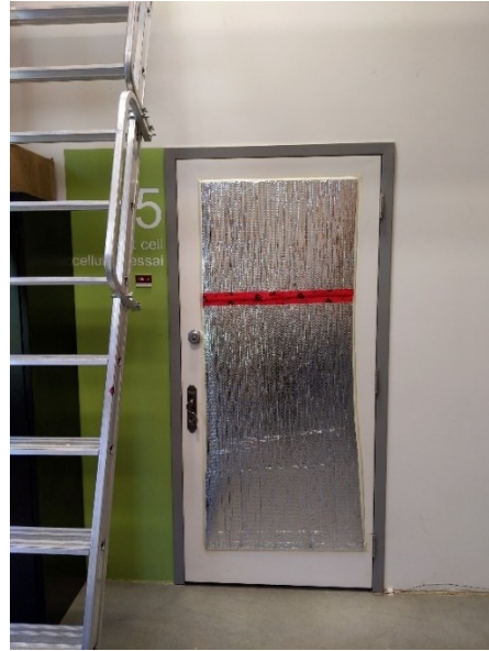
Figure 6.2.12: Reflective insulation applied to the interior test cell door
