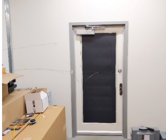
Figure 6.2.14: Black Bristol board insulation applied to the interior test cell door. Type-T thermocouples positioned on the door surface and near the wall.
