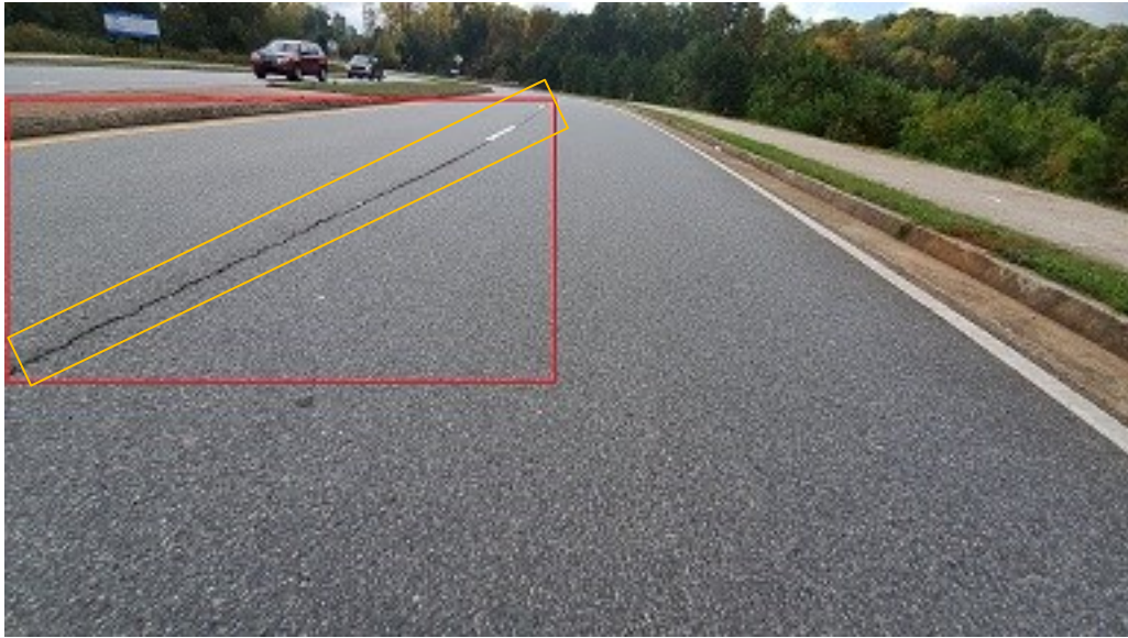
Figure 4-16 Comparing axis-aligned and oriented bounding boxes. Oriented bounding box comprises less part of background than axis-aligned bounding box
