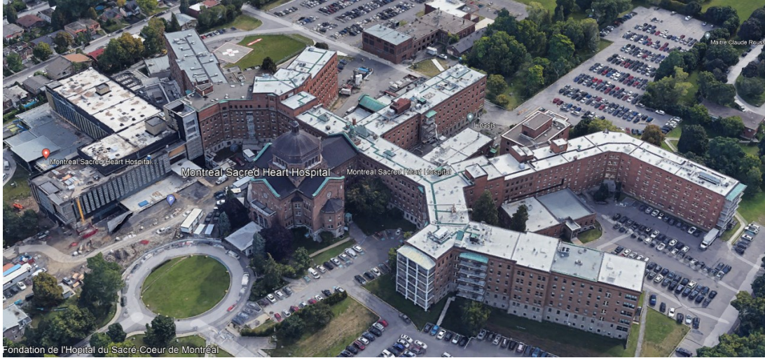
Figure 15: Snapshot taken from Google Earth of Hospital 1
