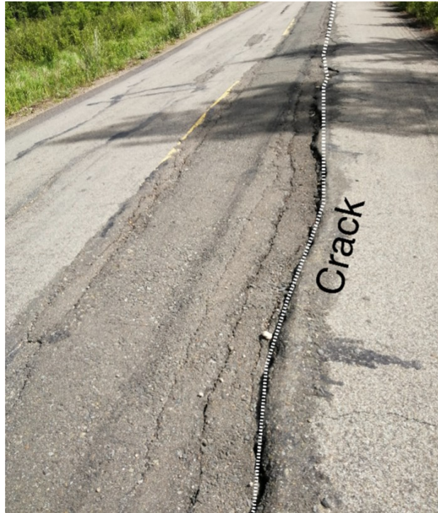
Figure 1.3 Shi-La Highway longitudinal cracks induced by the freeze-thaw cycle (Zhang et al., 2020)
