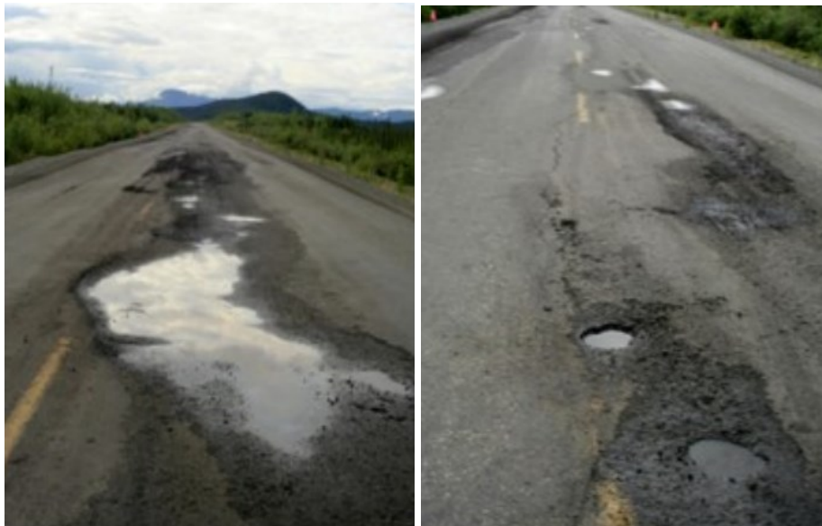
Figure 1.3 Shi-La Highway longitudinal cracks induced by the freeze-thaw cycle (Zhang et al., 2020)
