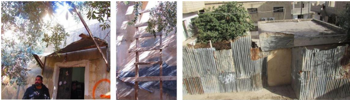
To the left and to the right, the use of zinc sheets provided once by the UNRWA as a roofing technique in different new ways: protection from rainwater at the home's entrance and as fencing material. In the middle, recycling wood to make handmade ladder
