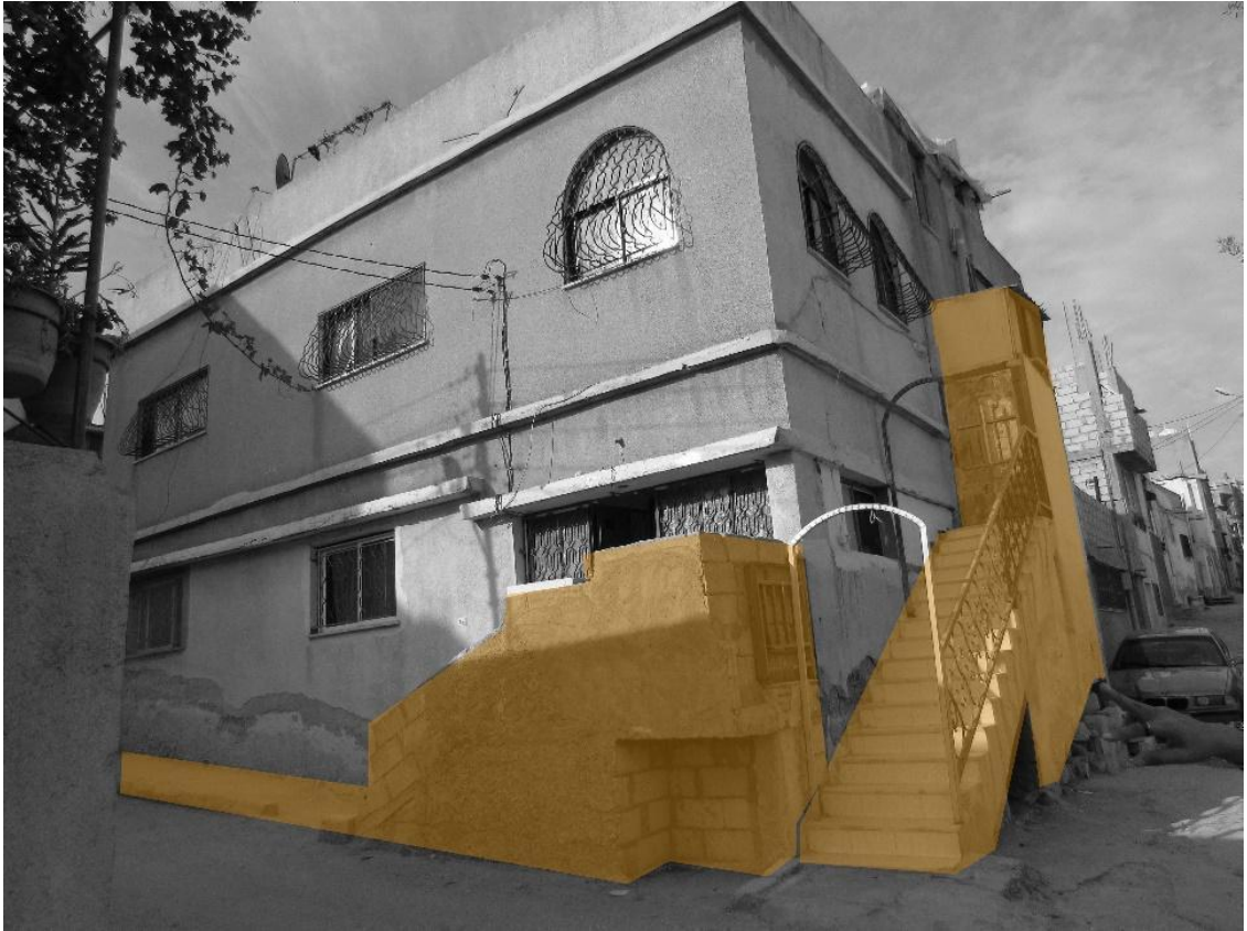
Figure 27. An edited photo of Mawali's home in Al-Husn camp showing, in orange, illegal structural additions, Irbid, Jordan (Alqub, 2021).
