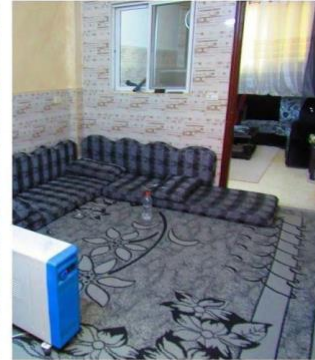
The use of ceramic tiles to treat wall mold and dampness
