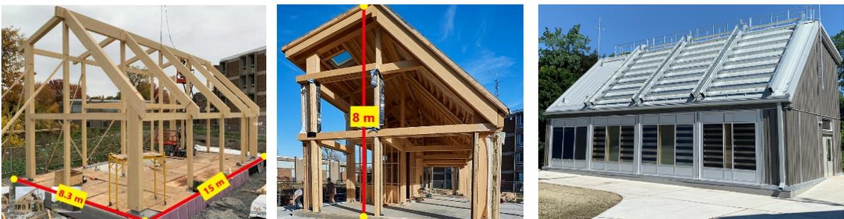
Figure 9. Future Buildings Laboratory in different construction stages
