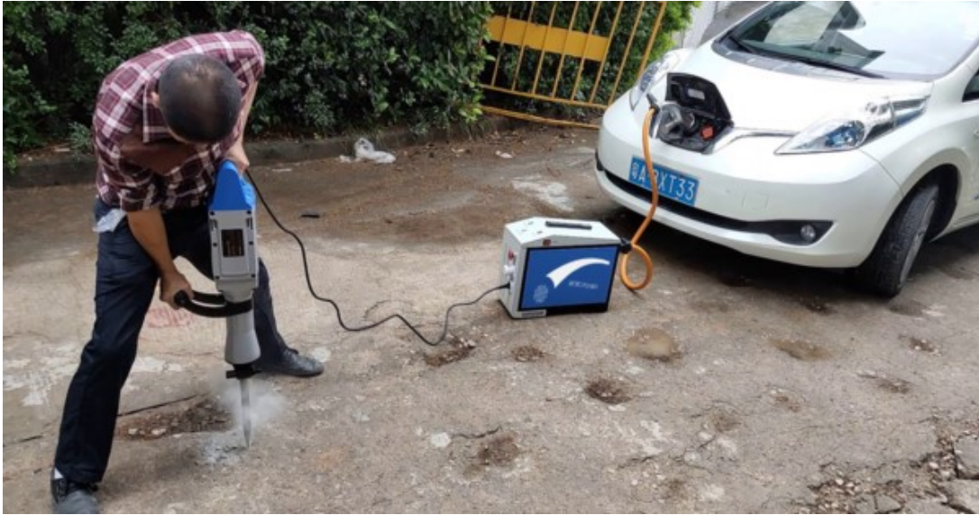
Figure 6-14 the car and Setec power charger connection [48].
