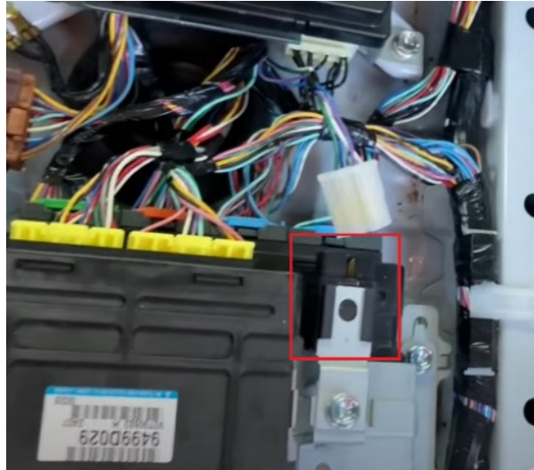
Figure 6-10 EV contactor control relay.
