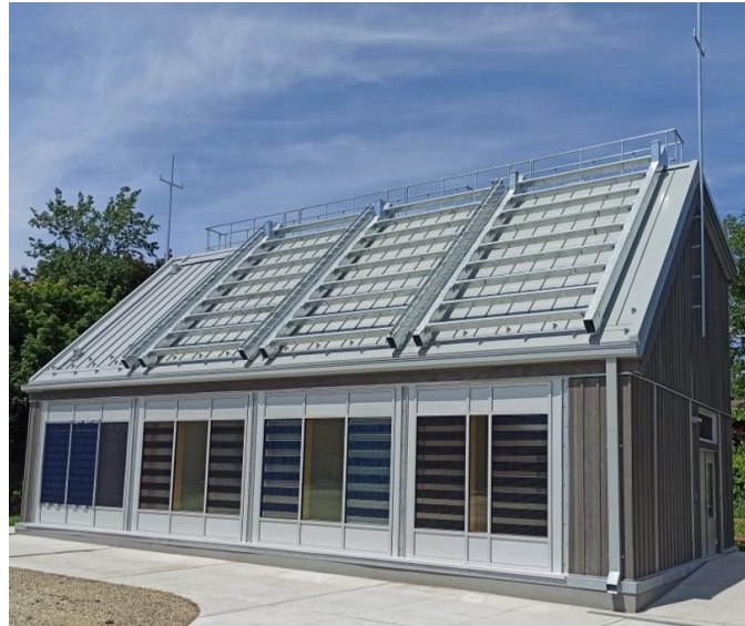
Figure 1-3: Future Buildings Laboratory (FBL).
