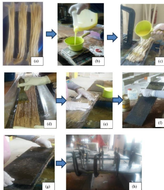
Figure 2.15: Fabrication process of natural composite plate; (a) Dividing fibers, (b) Weighting adhesive, (c) Pouring the adhesive, (d) Pressing the fiber, (e) Covering the mould with plastic, (f) Greasing the top plate, (g) Cover the mould with top plate and (h) Compressing the composite plate by clamps [93].
