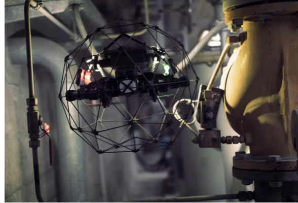
(b) Indoor Pipes and Valves Inspection [31]
