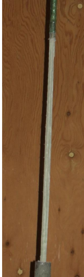
(b) Longitudinal cracks
