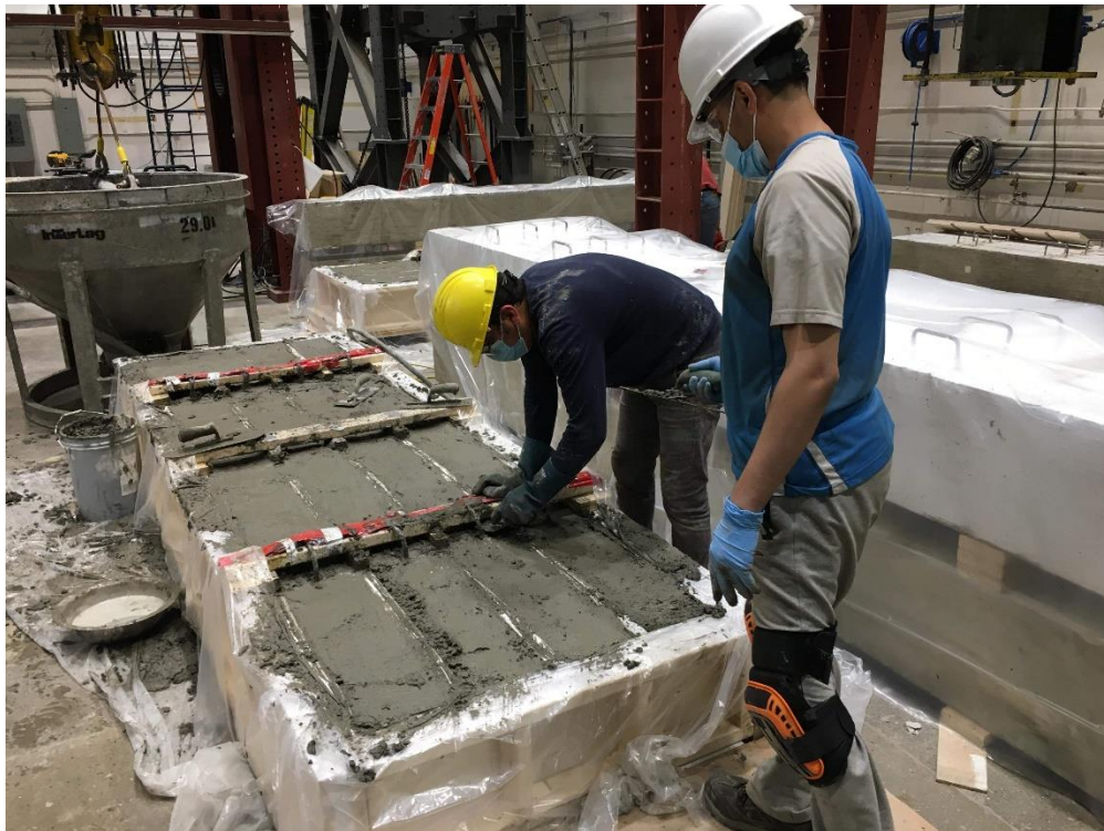
Fig. A.3 Finishing of the top concrete surface using trowels
