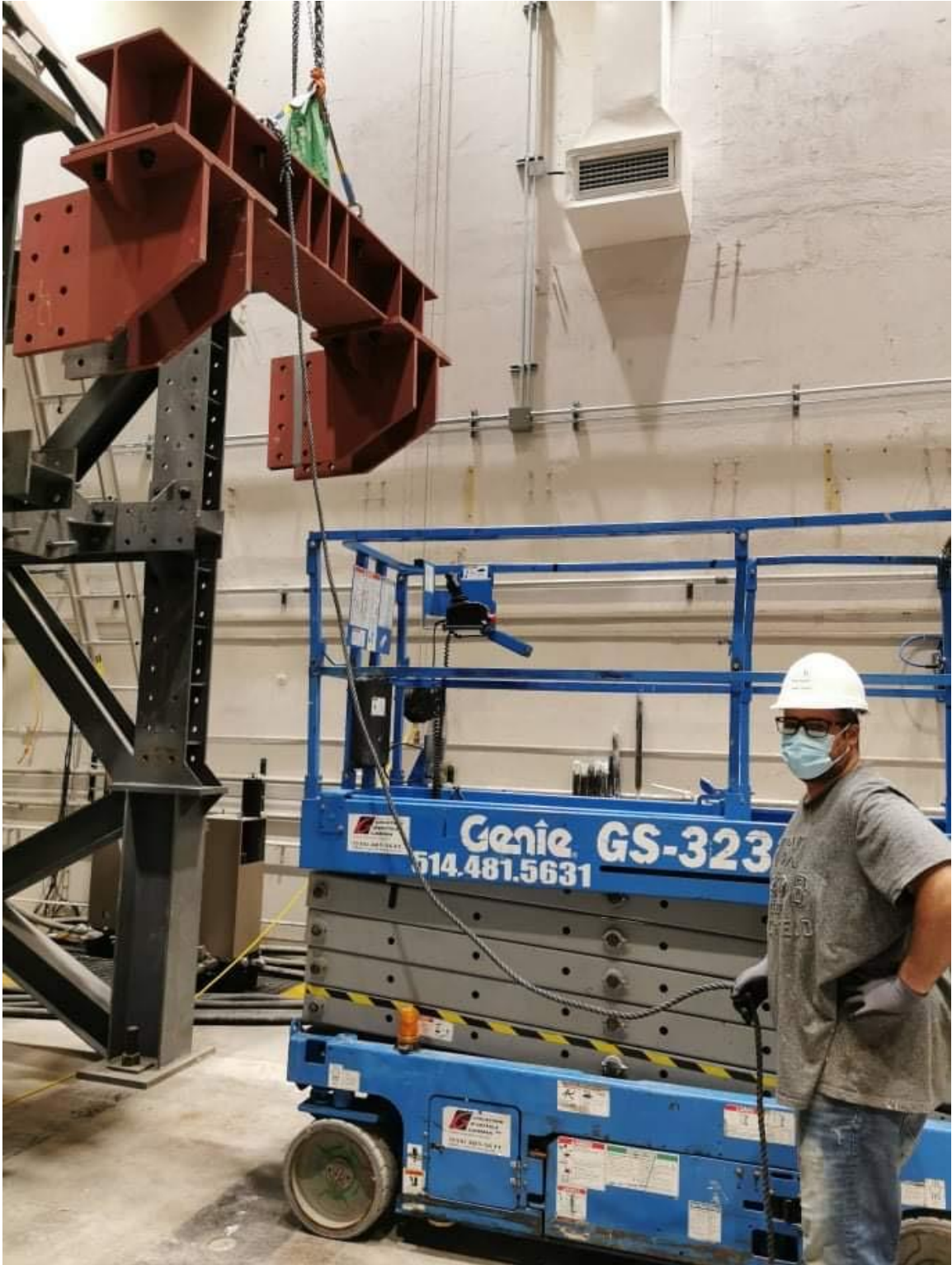
Fig. A.5 Construction of the testing frame
