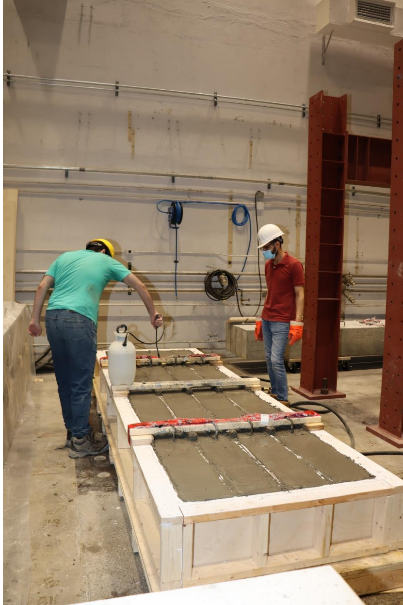
Fig. A.4 Curing of the poured concrete
