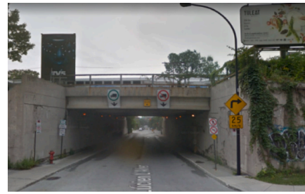
(b) Bridge 2: Lucian L'Allier Street
