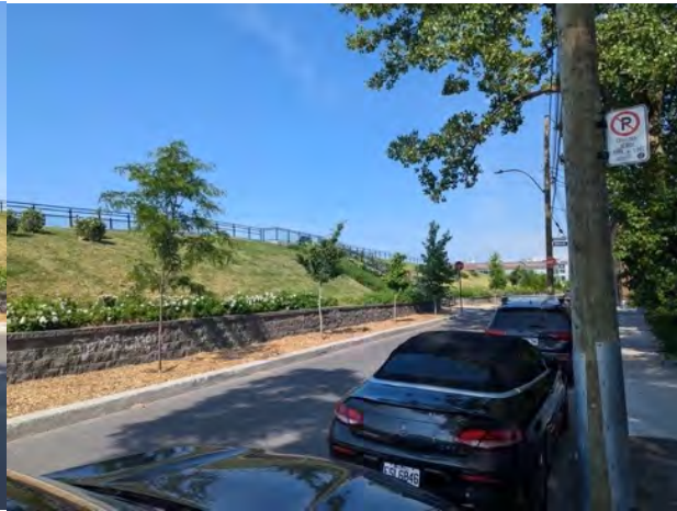
Figure 50: Sound wall continued. Demonstrating the relative length and height of the wall
