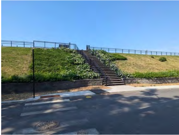
Figure 49: Sound wall built on Sebastopol
