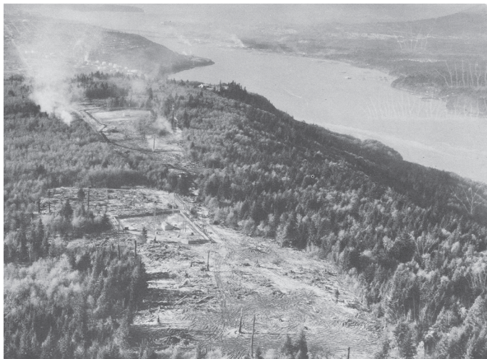
Site for the construction of the Simon Fraser University Burnaby campus, 20 November 1963. Photograph by George Allen
