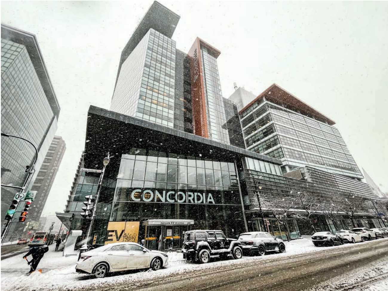
11.1 Engineering, Computer Science and Visual Arts Complex, west façade, corner Sainte Catherine and Guy Streets.
