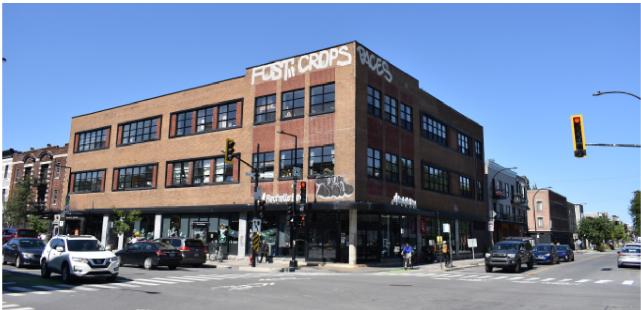
FIG. 13 THE INTERSECTION OF RACHEL ST. AND ST. DENIS BLVD IN MONTREAL
