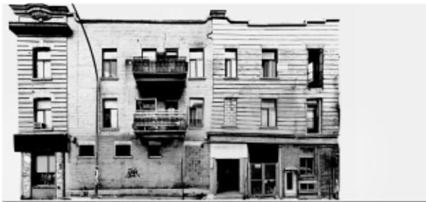
FIG. 23 TYPICAL PLATEAU BUILDING ALONG ST.LAURENT BOULEVARD
