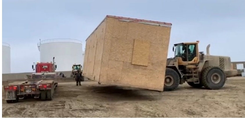
Fig. 39. Moving the pods from the shore to the assembly site
