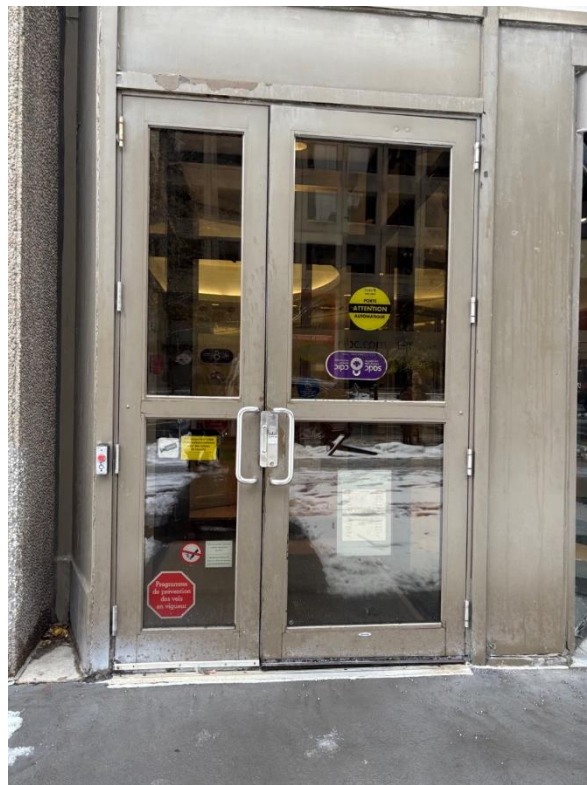
Figure 3.15 Case study (B) Exterior Door
