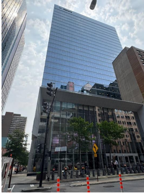
Figure 3.9 Case Study Type (A) Post-Code (New) Building
