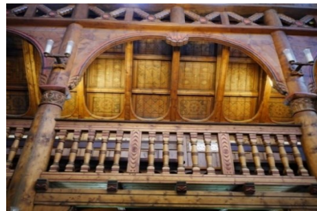
b) Well-maintained architectural building [4]
