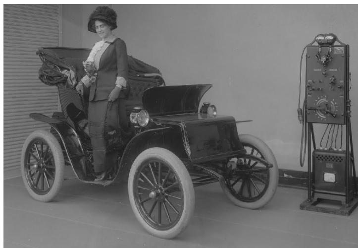
Figure 2.3: GE Mercury Arc Rectifier, circa 1912. An early electric car charger. [7].
