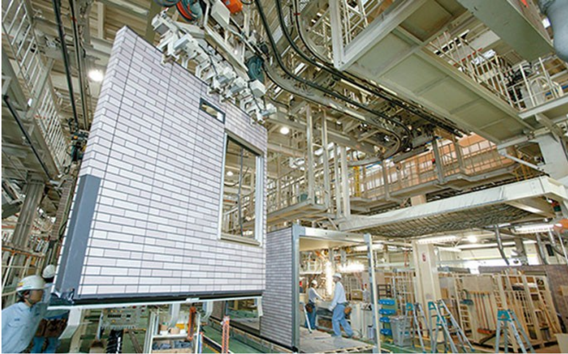
Figure 2-4 Example of modular construction in Sekisui House company (Adapted from (Modcoach, 2025))
